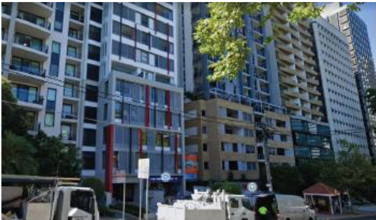
Figure 29 Recent Mixed-Use Tower Development along Miller Street
